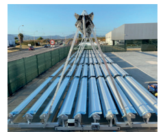
SOLPINVAP, Castellón (Spain)
